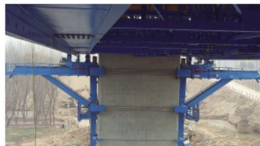
400 ton EAGLE PRO EL series hydraulic cylinders used in bridge building
